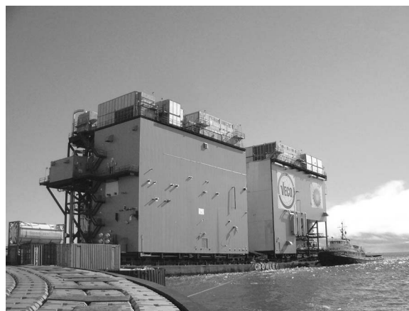
FIG. 2. Sealift barge 400 carrying two process modules, upon its arrival at Northstar Island’s southern dock on 10 August 2001. The Ocean-class tug Navigator can be seen alongside the barge on one side.
